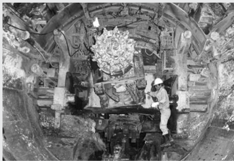
RIGHT: Mass Rapid Transit tunnels works being carried out in 1985.
