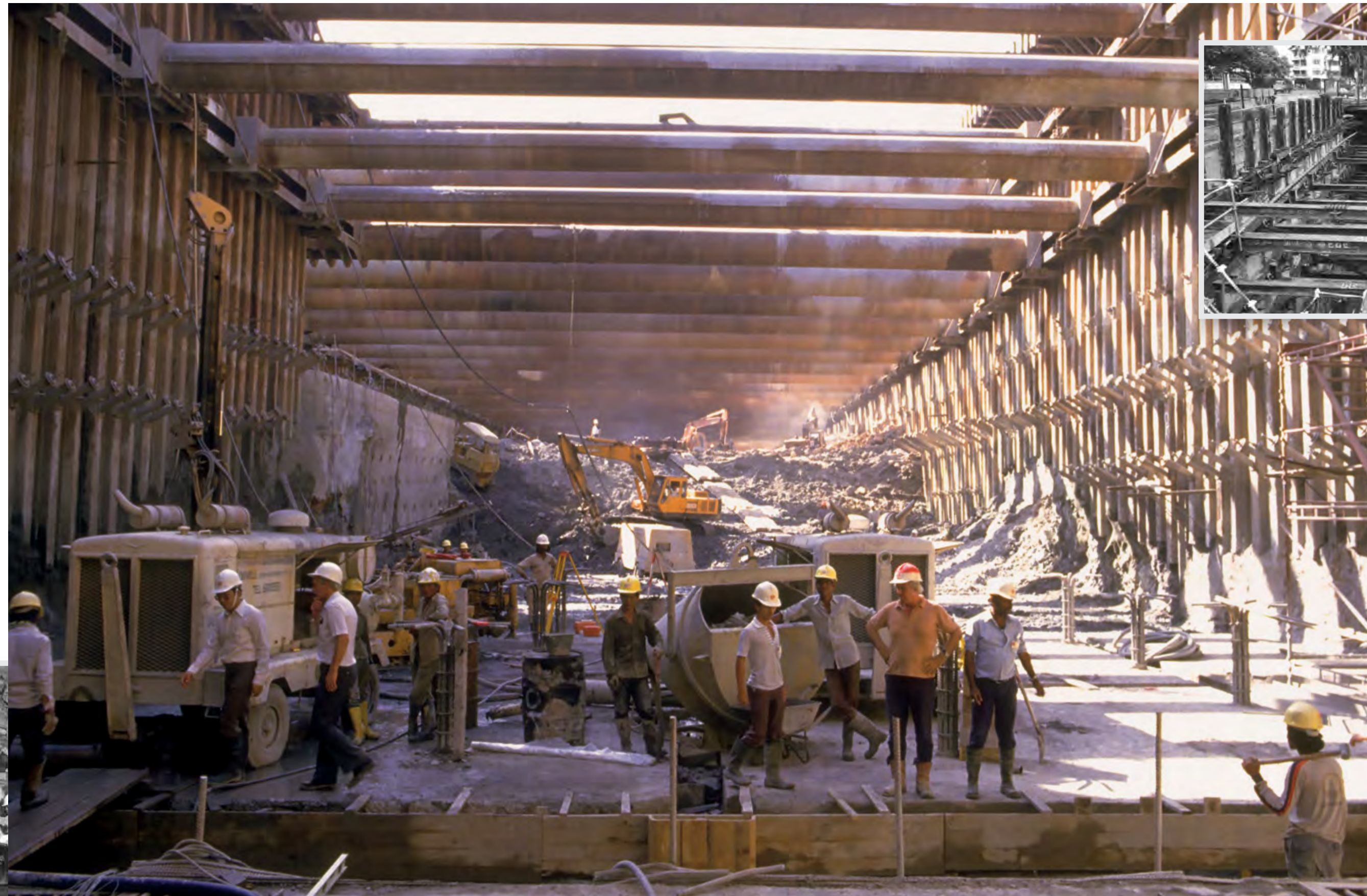
TOP: Steel beams and pillars provided the sturdy foundation for the Mass Rapid Transit tunnels.
